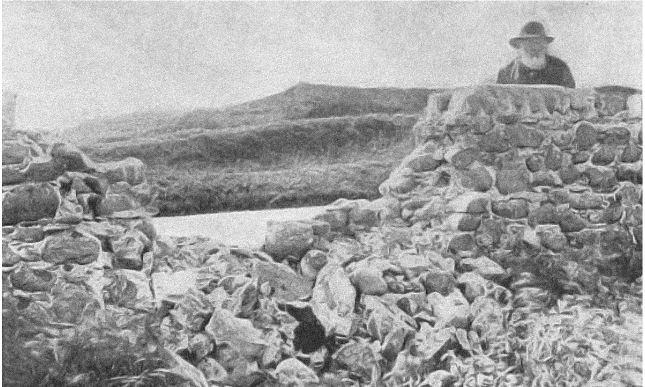
Fig. 19. Stone wall broken by lightning at Allonby, Cumberland.
