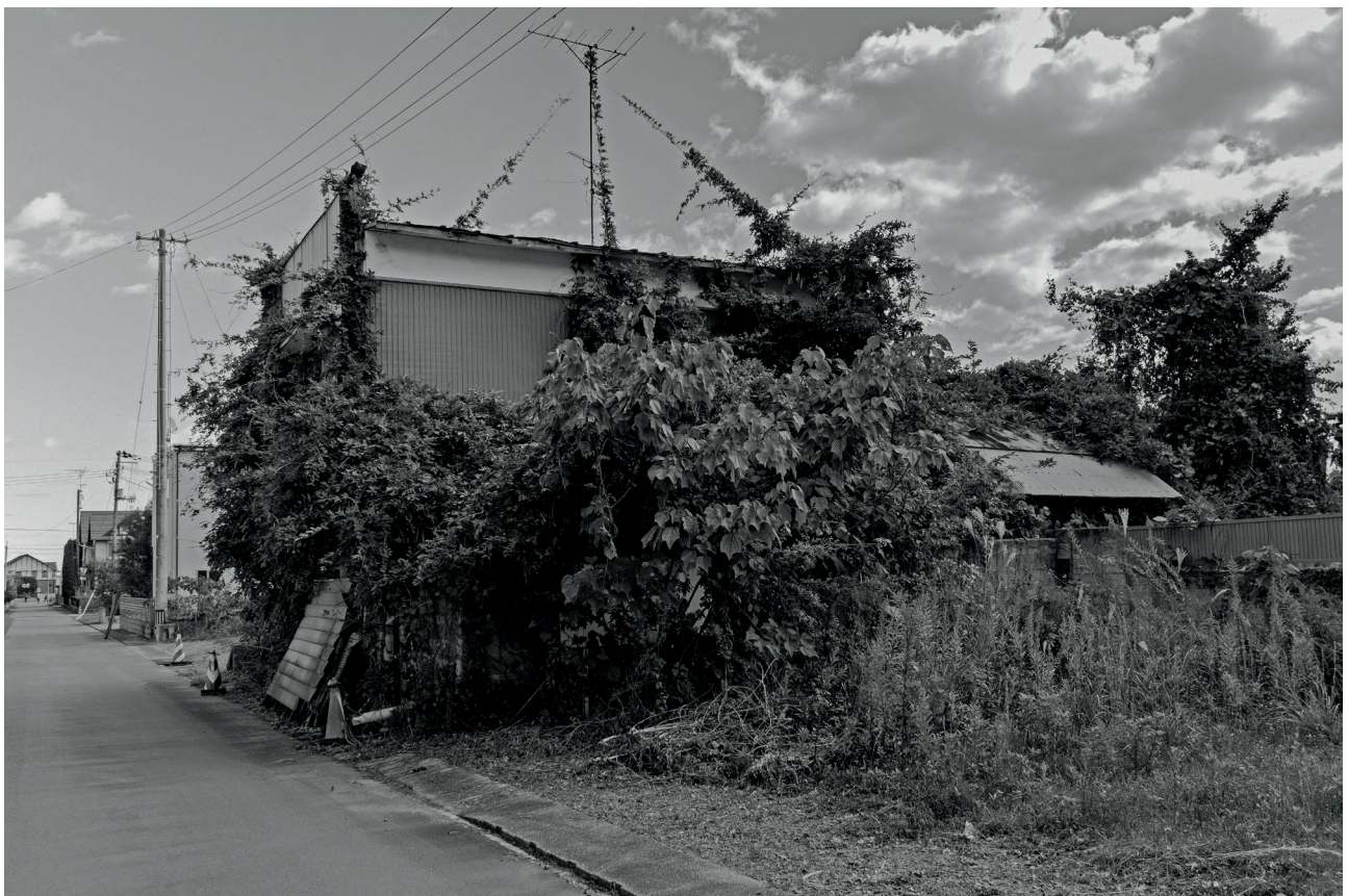
An overgrown building in central Namie.
