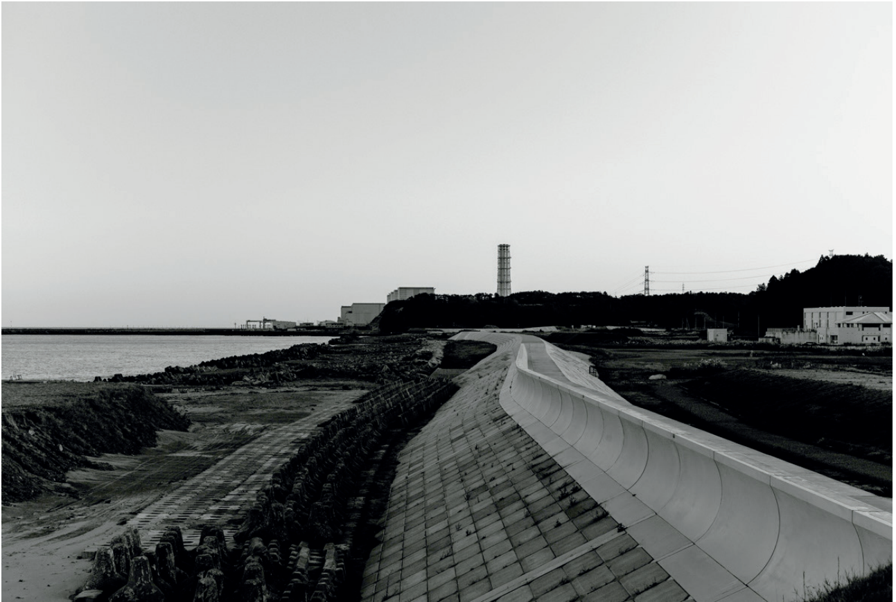
The coastline at Tomioka, with reinforced flood walls and the silhouette of the Fukushima Daini Power Plant in the background.
